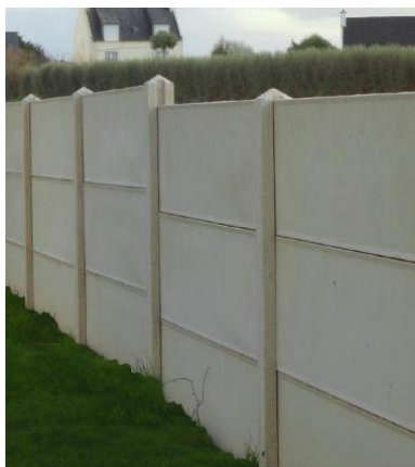
PLAQUES LISSES BETON MOULE
